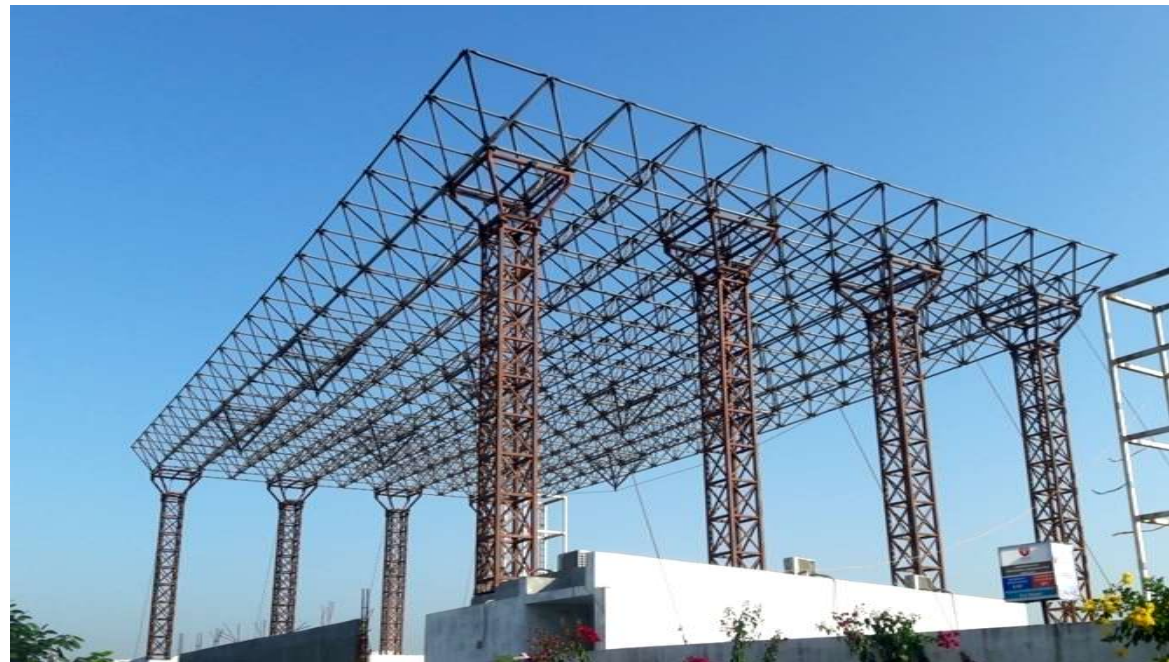
Private Stadium Roof Ankelshwar - Gujarat India
